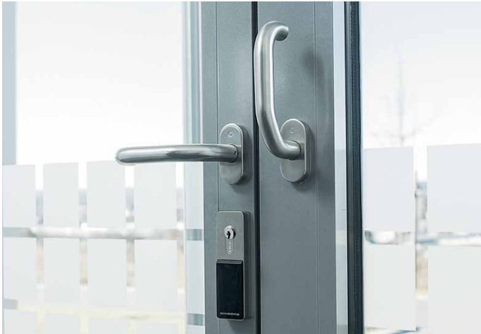
Surface fixed version – electronic module on the inside of the door.
