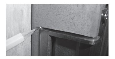
3. Peel the adhesive backing from tape on the back side of the appropriate faceplate. Remove the strike mounting screws. Hold the strike in position as marked on frame. Carefully position the faceplate onto the strike and secure to the frame.
