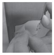
**3.** Carefully cut the frame inside the un-shaded area marked on the template. Install strike per installation instructions 08281280.
