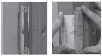
**2.** Peel adhesive backing and paste the folded template square to the frame.
