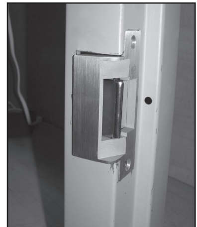
Ready to Secure: The strike is now in position ready to be secured by the two (2) 12-24 mounting screws.
