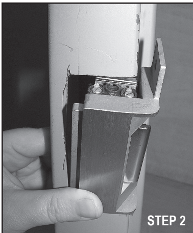
Strike Position: Rotate the strike into the frame. Note that the strike is angled slightly forward to clear the Pry-Guard.
