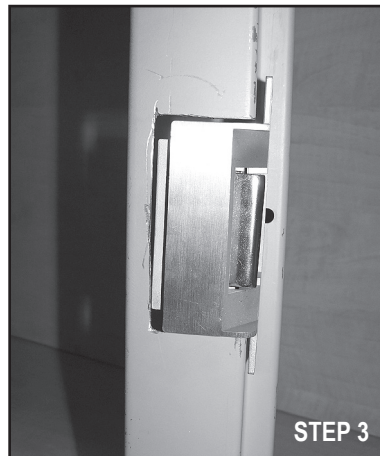
Final Push: Push the strike into the frame. The pry-guard should be behind the front lip of the frame.
