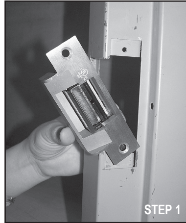
Initial Position: Place the strike as shown with the mounting tab located between the face plate and the insert.
