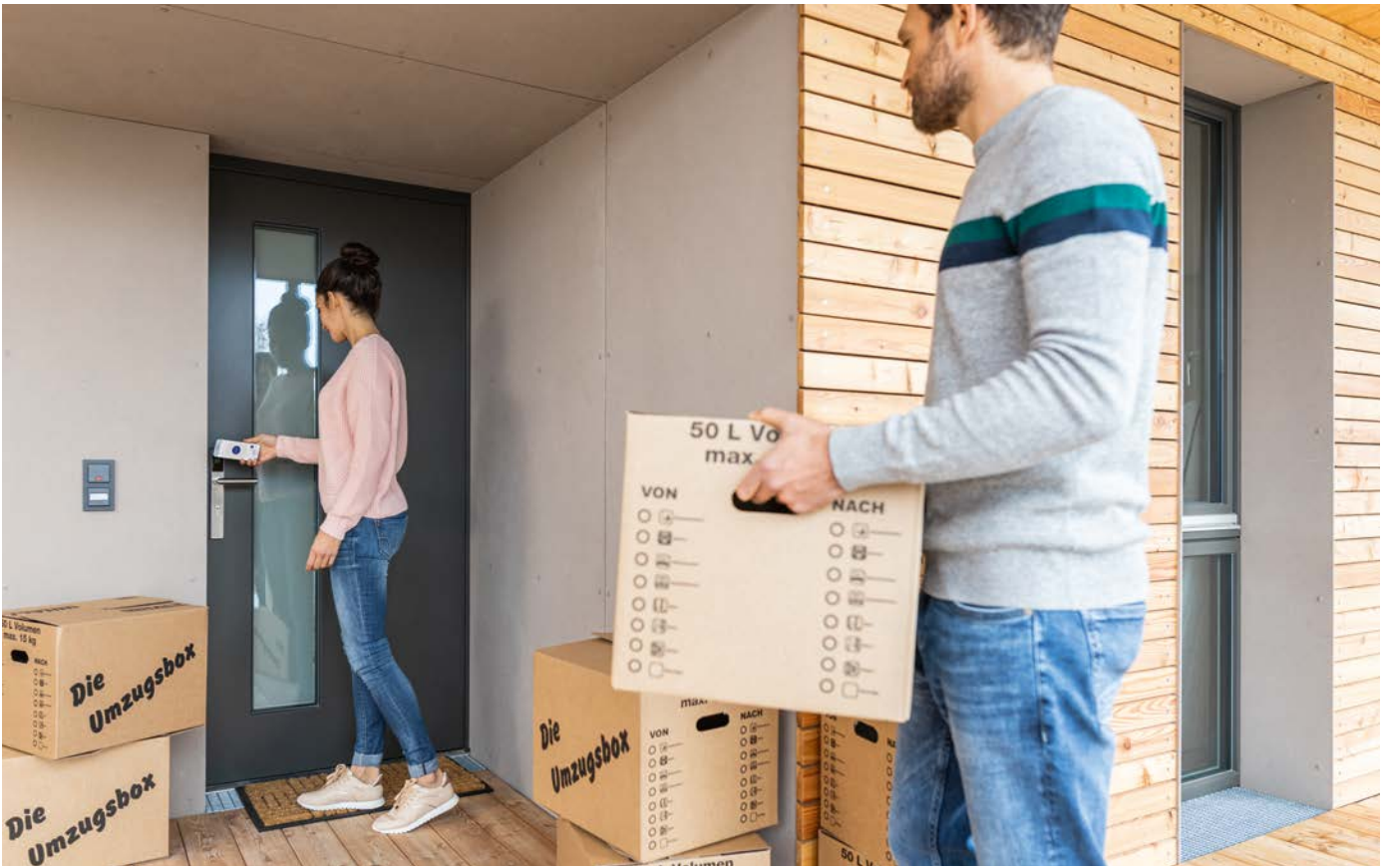
01 All apartments are equipped with an electronic door lock dormakaba c-lever.
