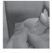
**3.** Carefully cut the frame inside the un-shaded area marked on the template. Install strike per installation instructions ISF2
